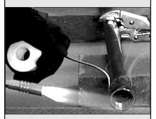
NOTICE: Do not solder pipes while they are attached to the water heater. The water heater's inlet and outlet connections contain non-metallic parts which could be damaged. The proper way to connect the water heater to copper water pipes is as follows:
