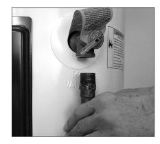
Figure 12 - Removing the T&P Relief Valve discharge pipe.
