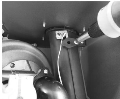
Figure 23: Exhaust port cap removal.
