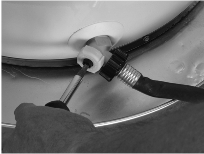
Figure 10 - Draining the old water heater.
