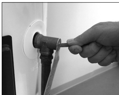
Figure 40 - T&P Relief Valve
