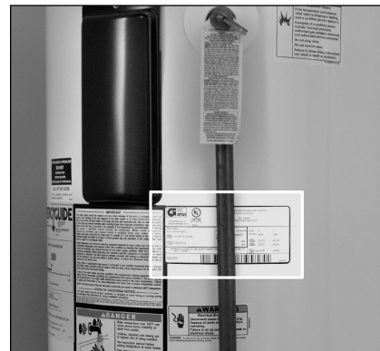
Figure 20 - The water heater’s electrical requirements can be determined from the data plate.
