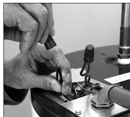
Figure 21 - Connecting the electrical wires.
