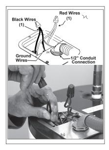
Figure 19 - Connecting the electrical wires.
