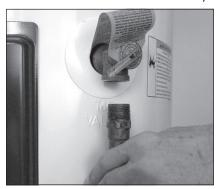
Figure 11 - Removing the T&P Relief Valve discharge pipe.
