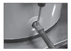
Figure 10 - Draining the old water heater.
