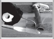
NOTICE: Do not solder pipes while they are attached to the water heater. The water heater's inlet and outlet connections contain non-metallic parts which could be damaged. The proper way to connect the water heater to copper water pipes is as follows:
