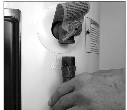
Figure 12 - Removing the T&P Relief Valve discharge pipe.
