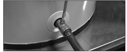
Figure 37 - Drain Valve.
