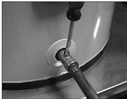
Figure 11 - Draining the old water heater.
