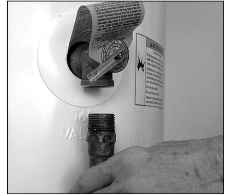
Figure 21 - Removing the T&P Relief Valve discharge pipe.
