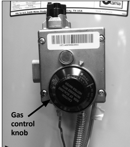
Figure 17 - Turn gas control/temperature knob OFF.
